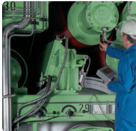
Registering vibration levels
